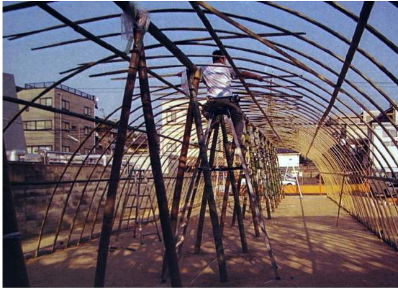
Figure 13: Building Process of the Bamboo Greenhouse (Bamboo Greenhouse, 2011)
